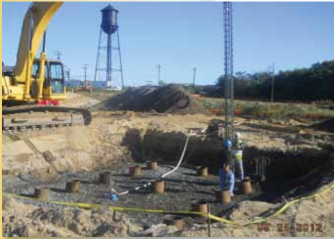
Setting of rebar cage within steel pipe pile for bridge foundation
