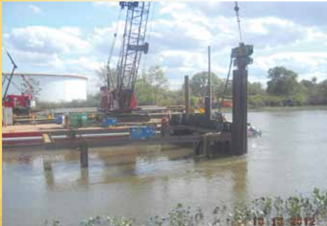
Installation of steel sheetpile to create bridge cofferdam
