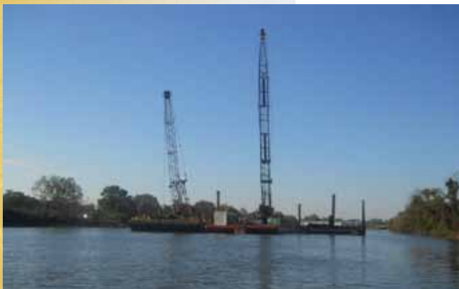
Commencement of bridge infrastructure: view of Mantua Creek looking upstream (south) - AP Construction's barge mounted cranes
