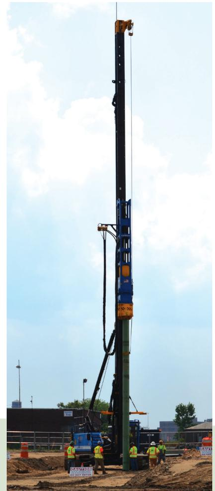
*THE HOLTEC GROUNDBREAKING—At the conclusion of the ceremonial ground-breaking this pile-driving machine shown at right drove the first of 4,000 concrete-filled steel piles into the ground. The piles will become the foundation of the developing Holtec complex.*
