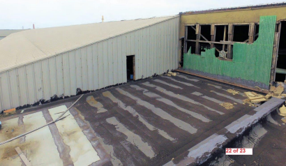
2. GUTS AND SIDING REPLACEMENT LOOKING NORTH
