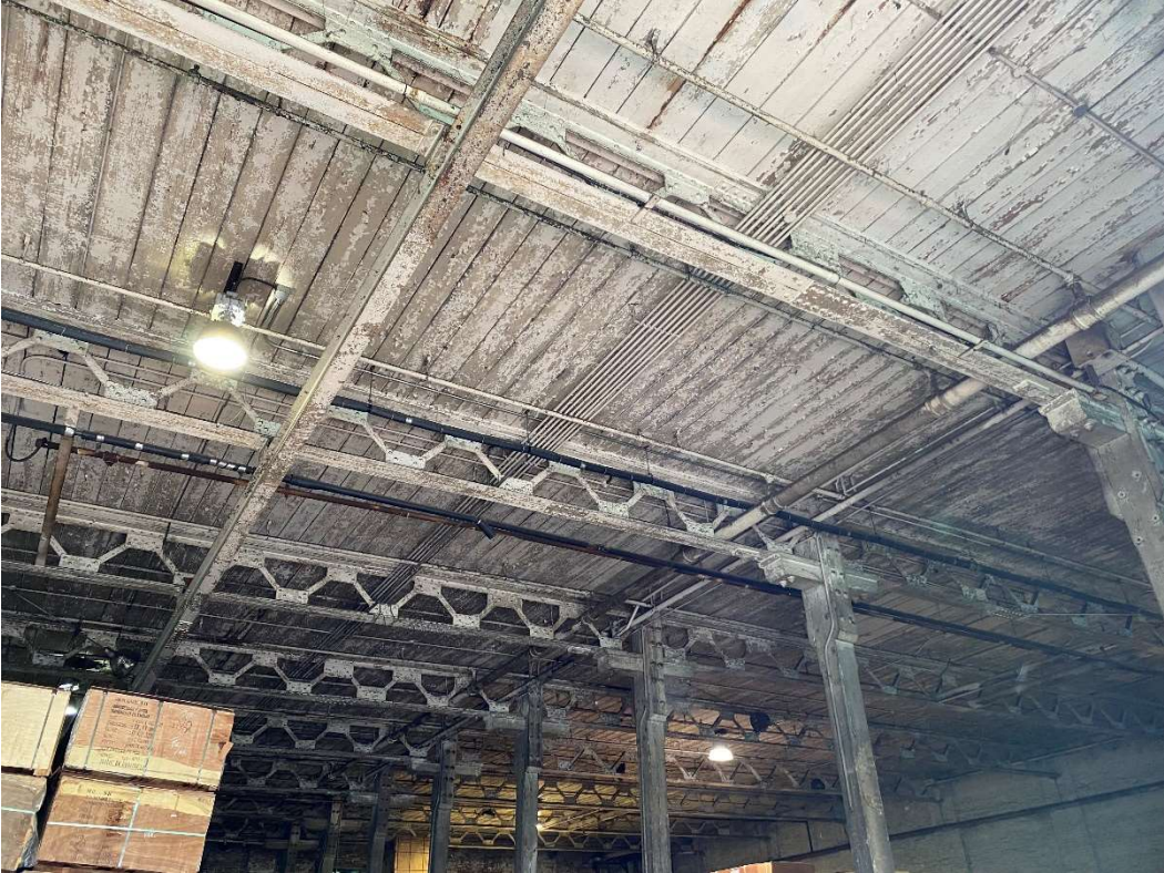
Photo 9: Interior – Building F
