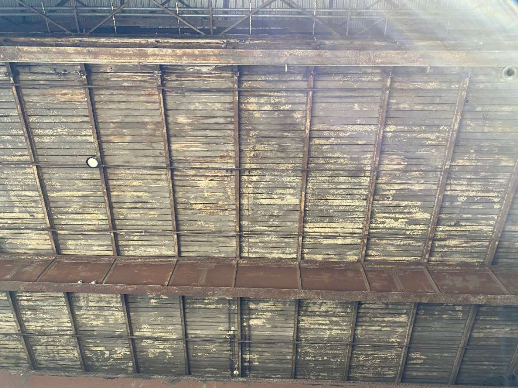
Photo 8: Interior – Building D
