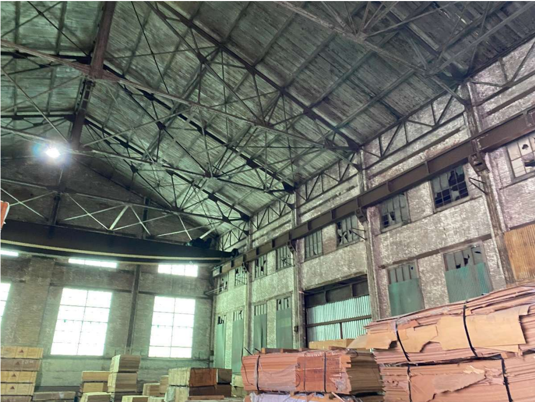
Photo 12: Interior – Building A-2
