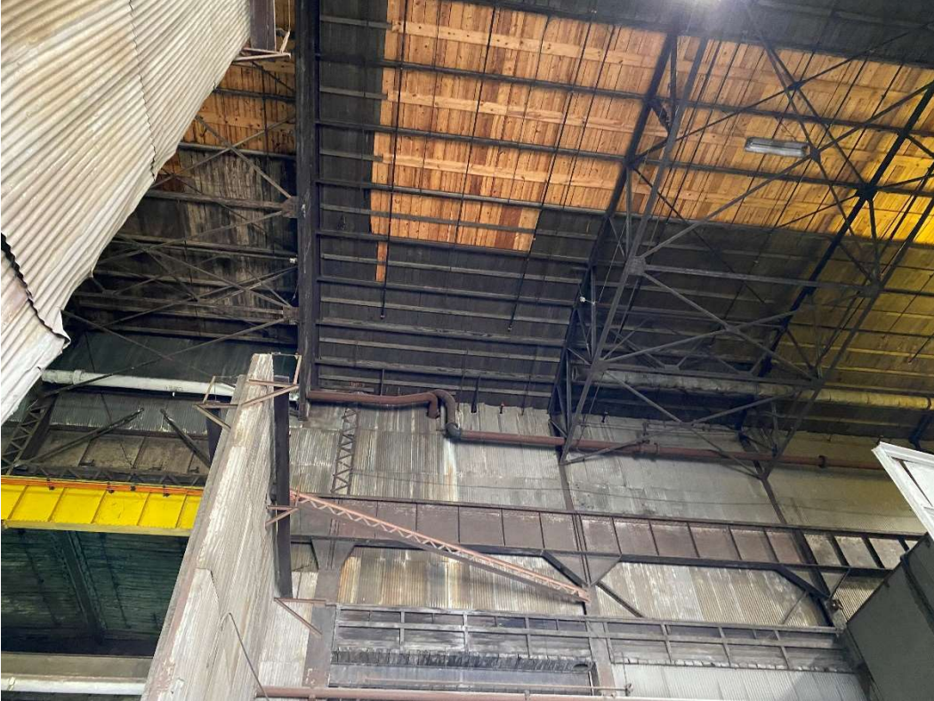
Photo 1: Interior – Building B
