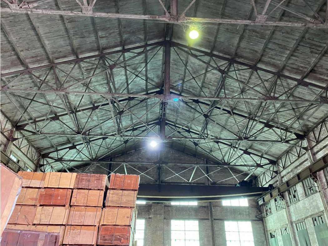
Photo 11: Interior – Building A-2
