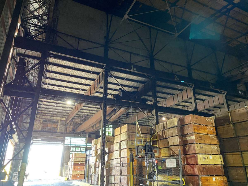
Photo 6: Interior – Building C/D
