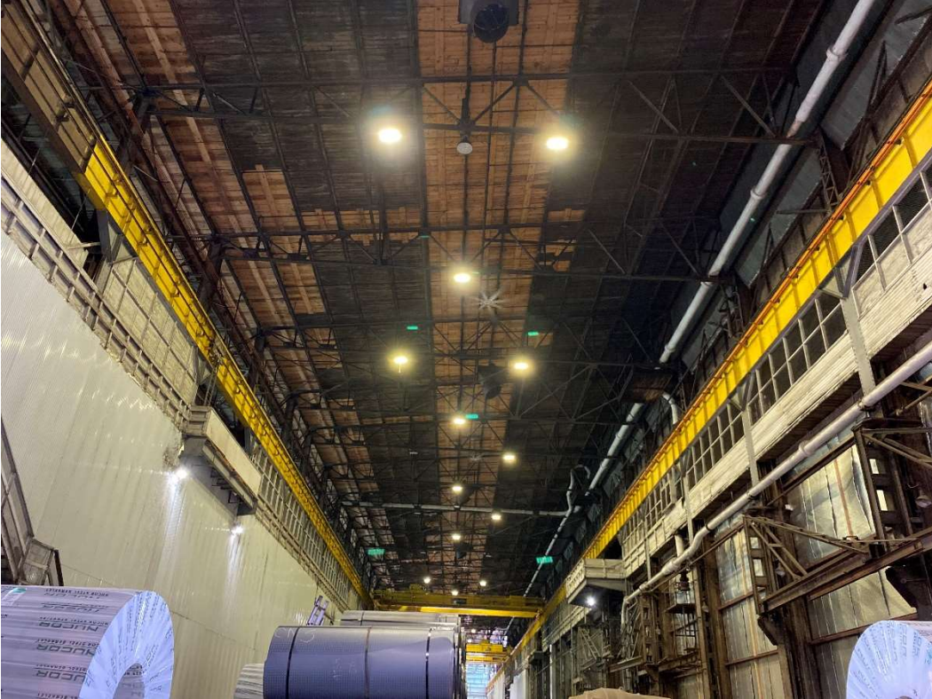
Photo 3: Interior – Building B
