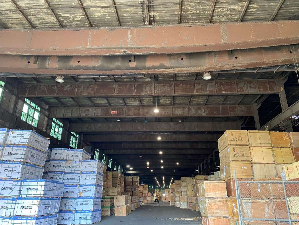
Photo 7: Interior – Building D
