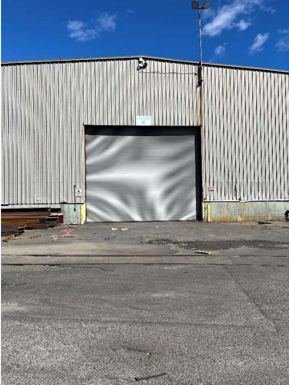
BUILDING E SOUTH END ROLL-UP DOOR
