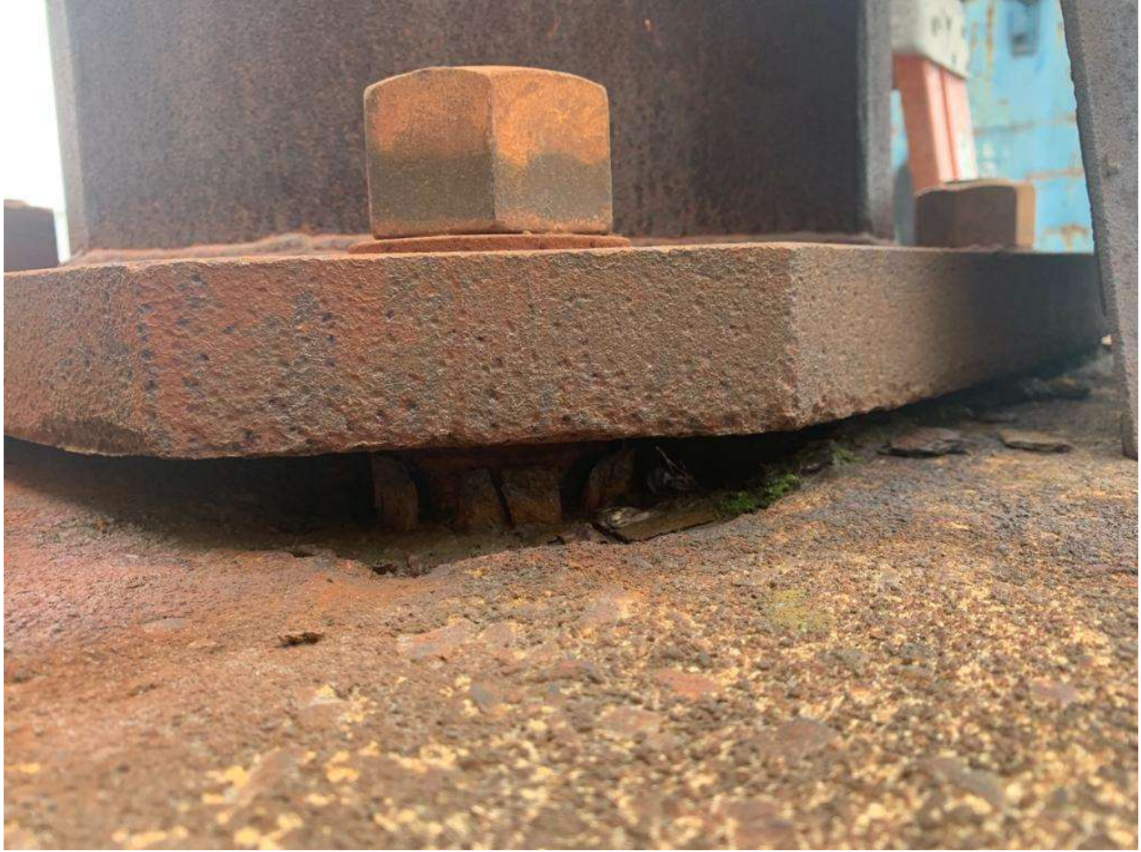
LIGHT POLE # 6 BASE
