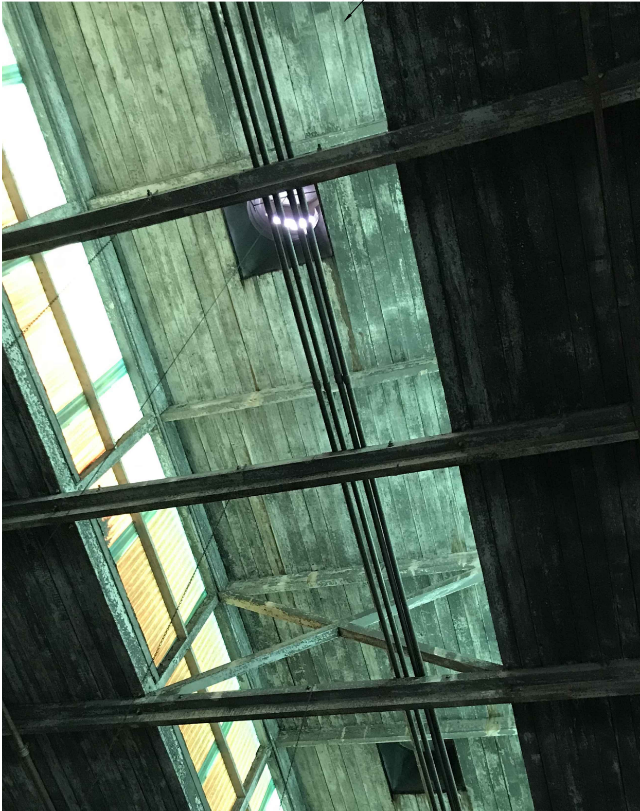
EXISTING DOGHOUSE & CROSS BRACING
