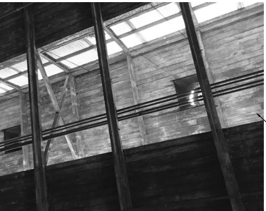
EXISTING DOGHOUSE & CROSS BRACING
