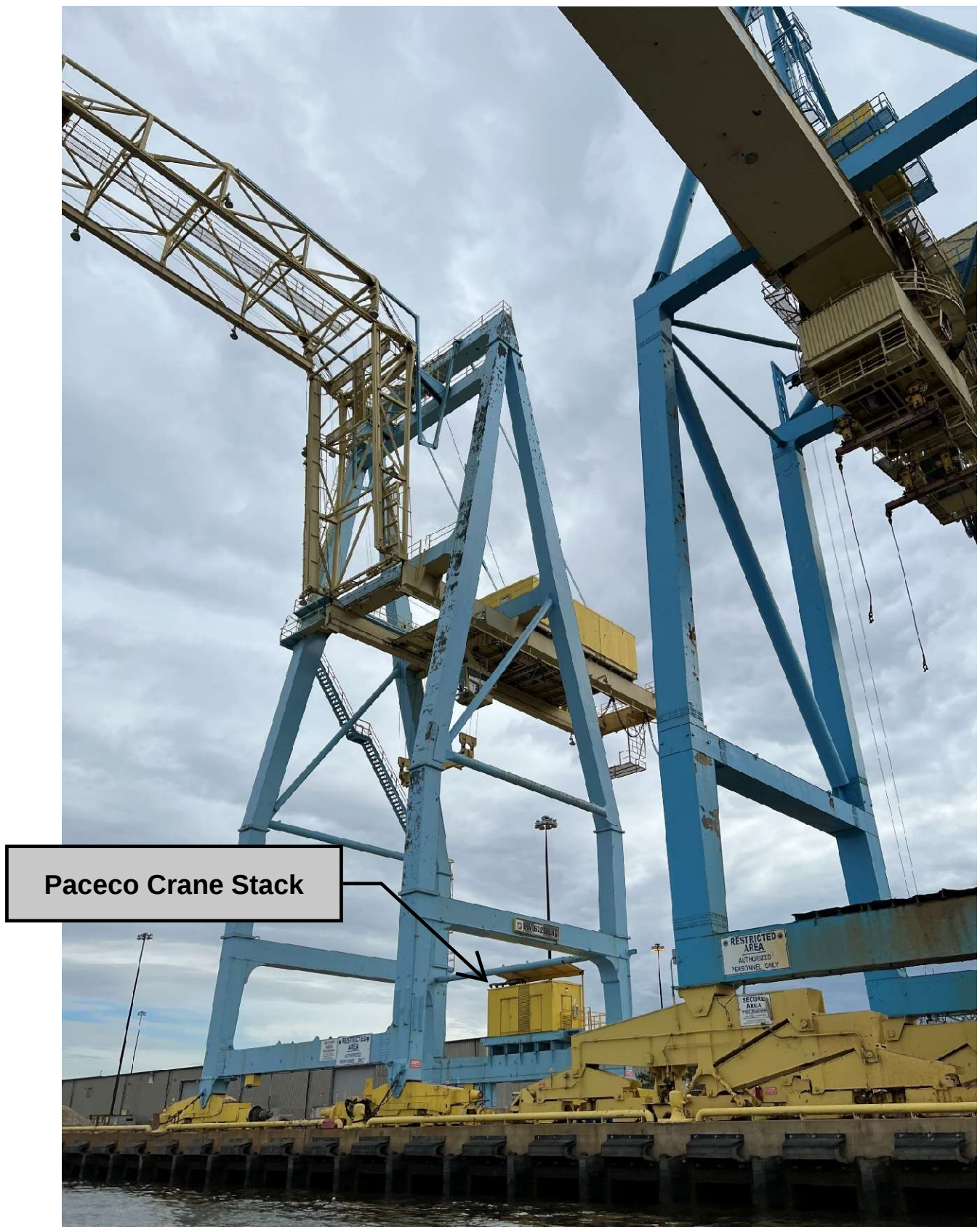
Paceco Crane on the left - Kocks Crane on the right
