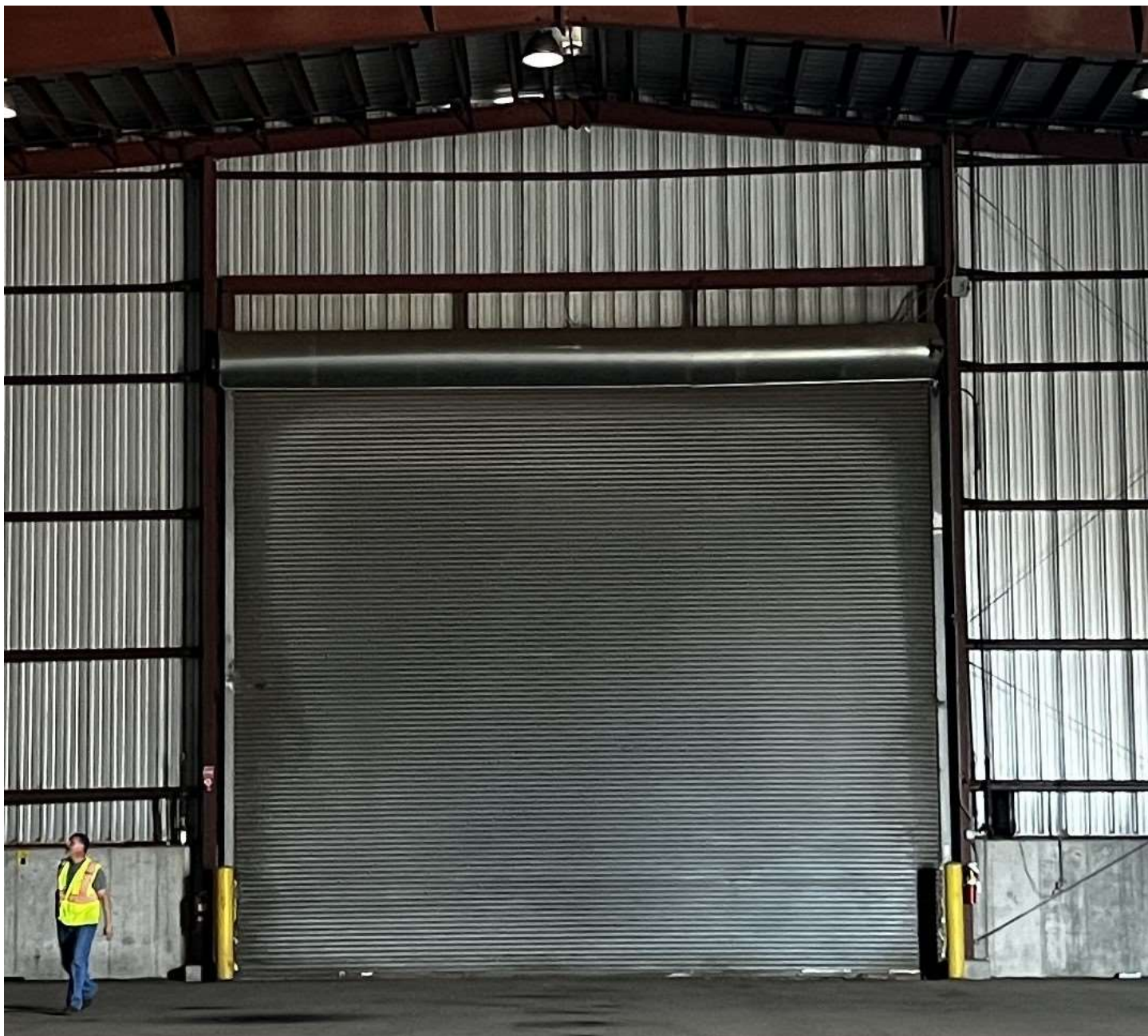
Building F2 West Door - Interior view
