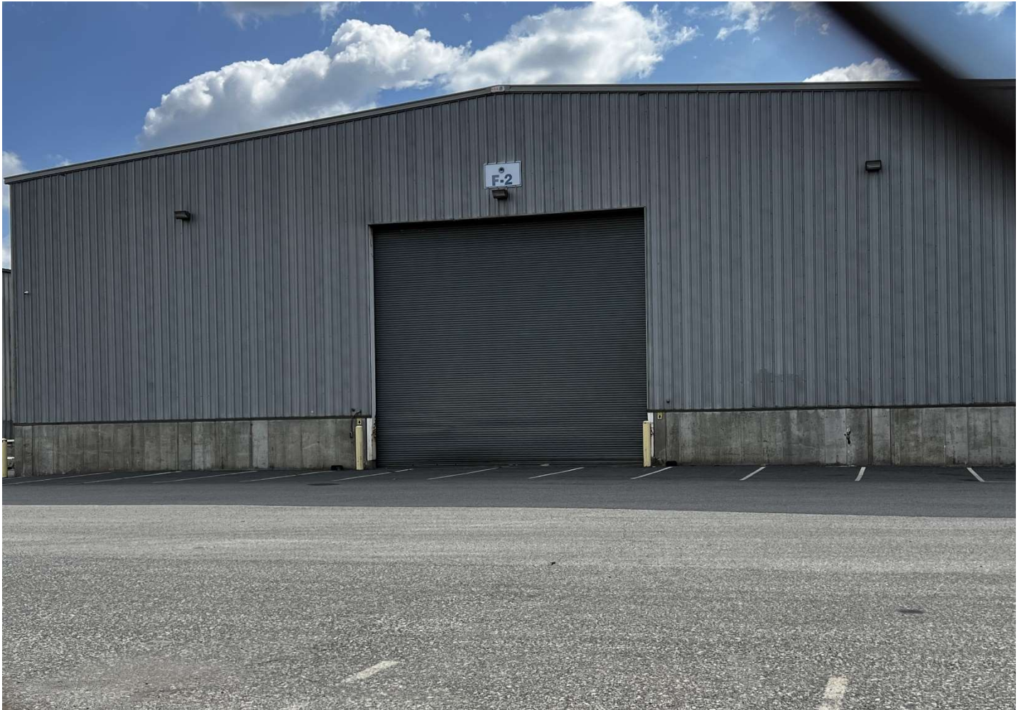
Building F2 West - Exterior View
